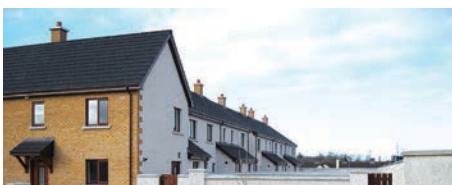
Social Housing Installation Co. Louth, Ireland
