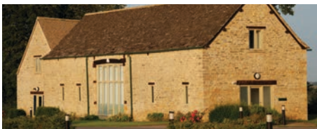
Barn Conversion Wing, England
